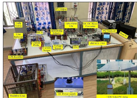
Fig. 7. Overall experimental setup of grid-tied solar PV system
