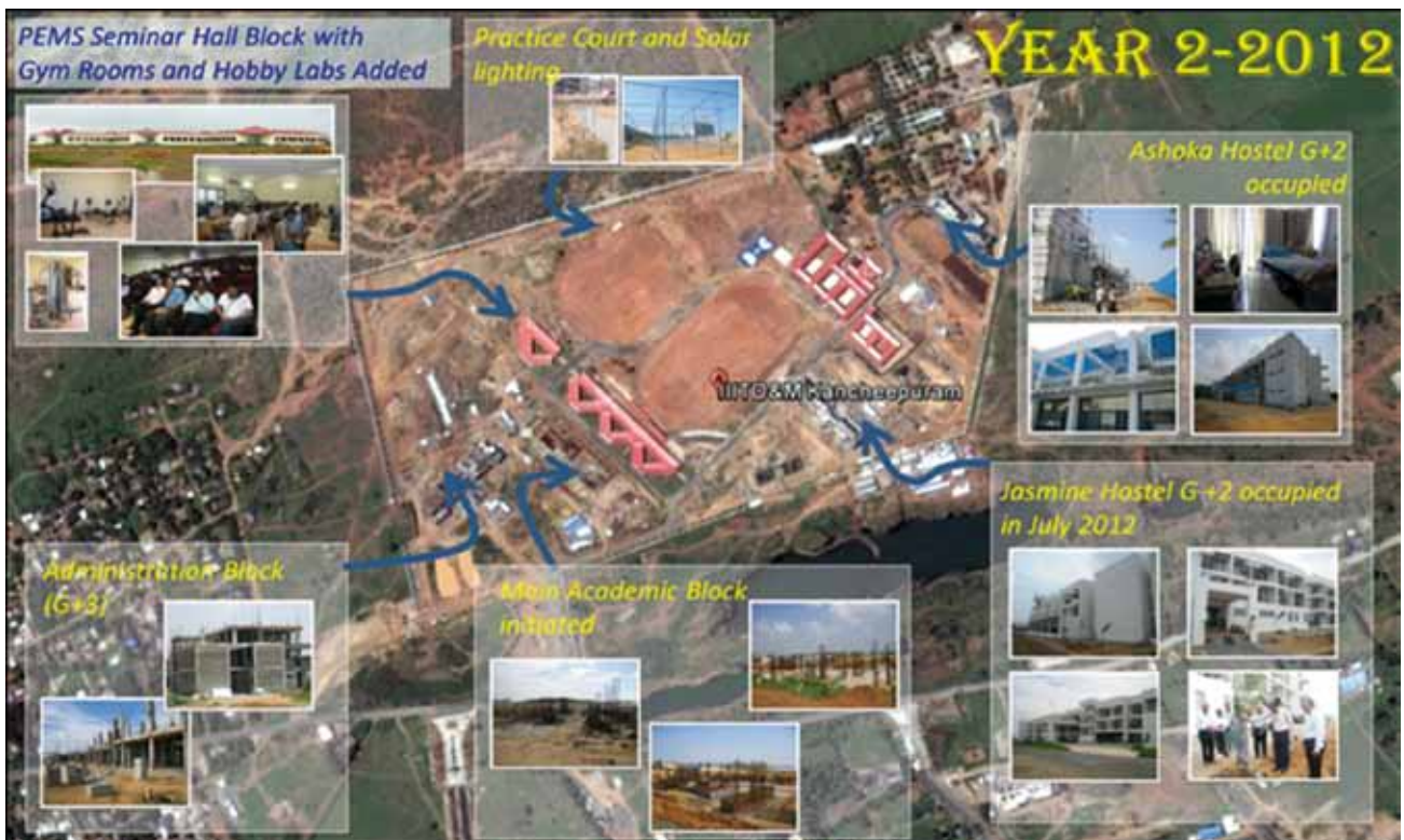
Phase I of the Permanent Hostel Buildings were constructed
